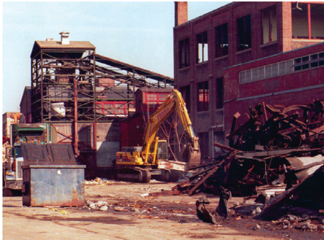
Demolition of the HB Smith Boiler Company, Westfield. | Photo provided by Tighe & Bond
