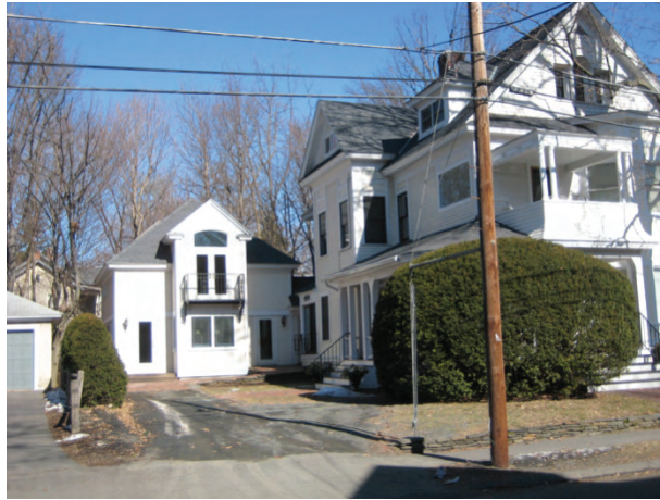
Example of a detached accessory dwelling unit in Northampton, MA. Source: Dillon Sussman
