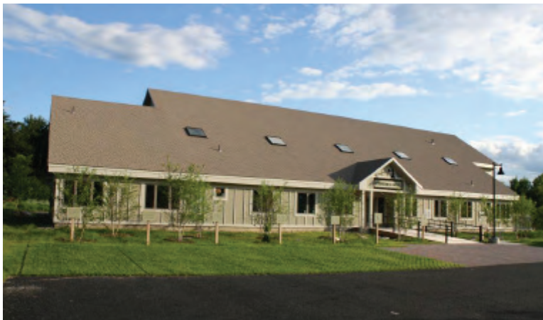
Figure 2: New England Environmental, Inc. with porous asphalt drive in foreground and grass paver parking stalls in middle ground | Courtesy: Mickey Marcus, NEE
