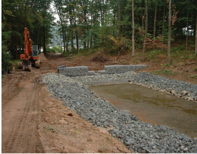
Congamond Lakes Restoration Project, Southwick
