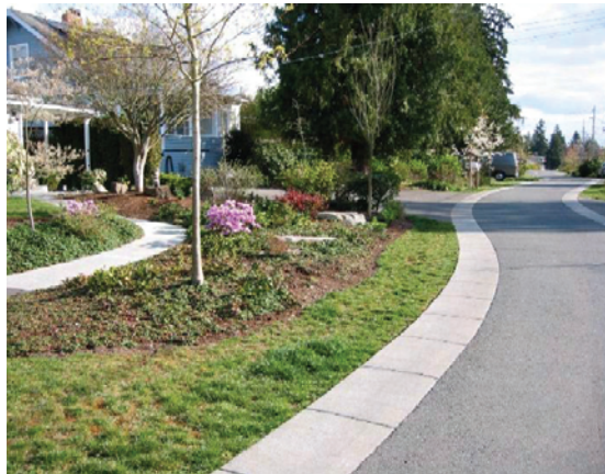
Streets designed without curbs allow water to drain into natural systems, such as gardens
