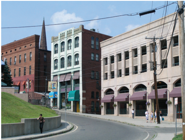
Northampton Parking Garage
