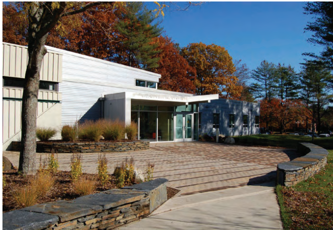
New 6,700 square foot addition to the Jerome Liebling Center for Film, Photography and Video, a part of the Arts Complex at Hampshire College.
