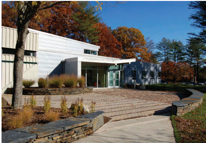
New 6,700 square foot addition to the Jerome Liebling Center for Film, Photography and Video, a part of the Arts Complex at Hampshire College.
