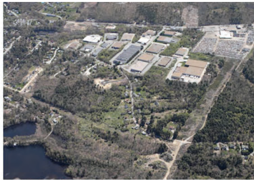
Aerial view of the Star Container Corporation complex
