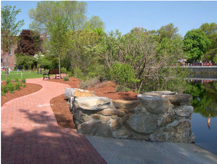
Pervious pavers used for the walkways at Riverfront Park in Orange, MA.
